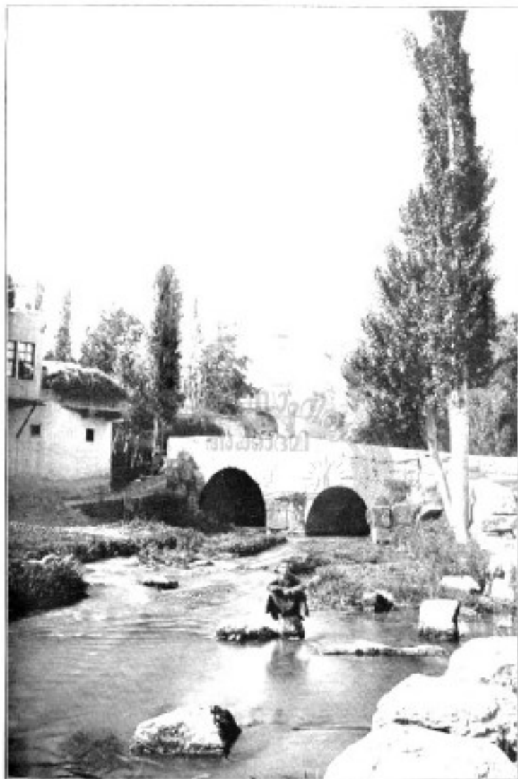
FIG. 1. BRIDGE OVER THE KIZILIA ST.
